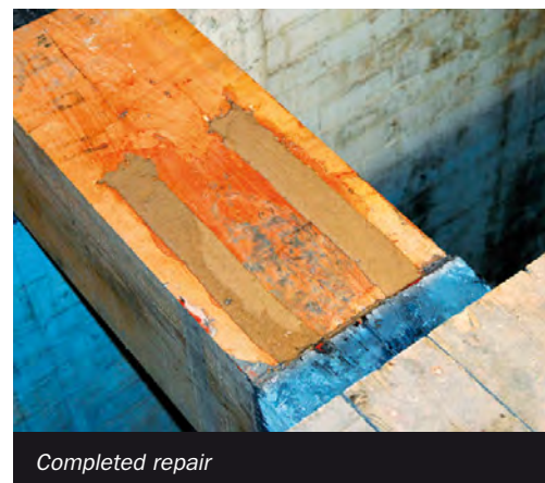
Steels fixed into existing timber using Trifix
