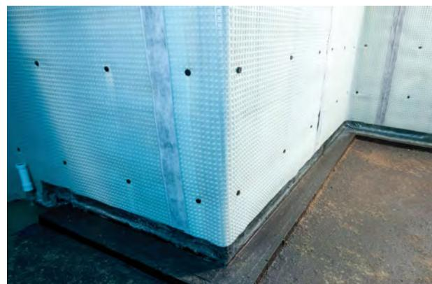
*Engineering brick detail housing Aqua Channel, with non-return odour resistant valve awaiting fitting (far left)*
