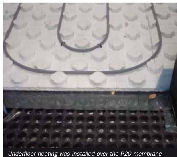
*Underfloor heating was installed over the P20 membrane*
