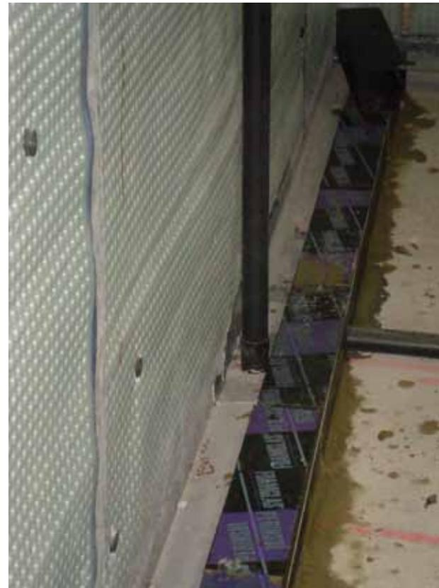
*The cavity drain system in the upper basement lever was gravity drained down to the system below*
