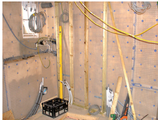
Areas waterproofed with Platon P8 membrane were battened and boarded.
