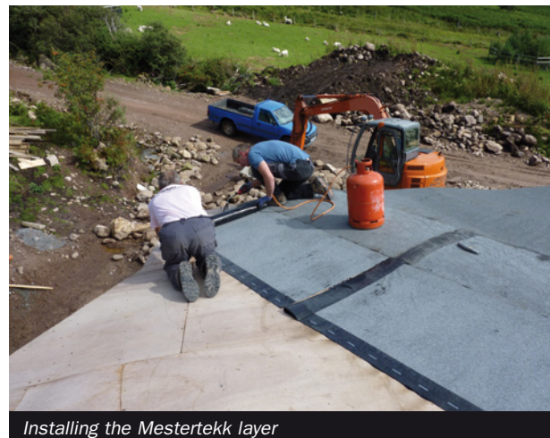
Sarking prior to green roof construction
