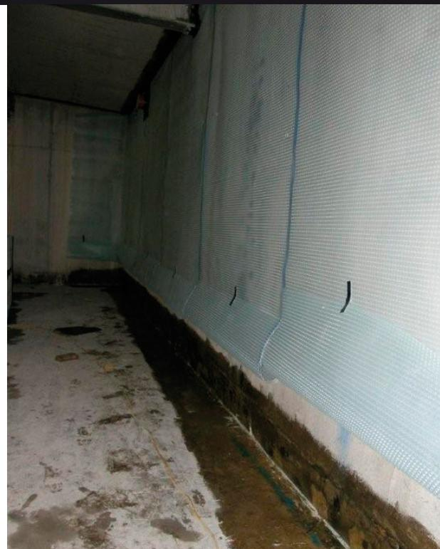
*Reinforced concrete wall floor junction tanked with Trimol 40 epoxy resin, before installation of blockwork upstand to house Aqua Channel drainage detail*
