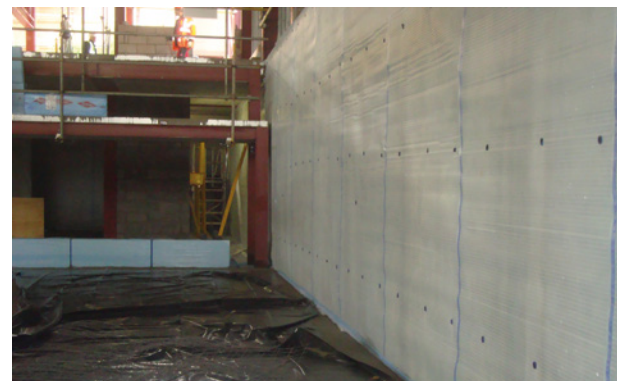
Platon Multi was installed to the walls
