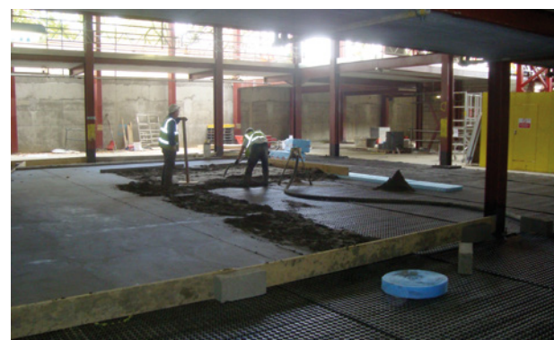
A screed can be applied directly to cavity drain membranes laid on the floor
