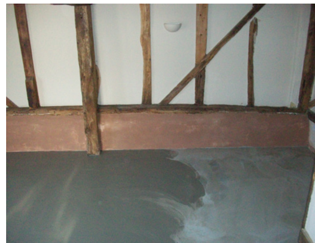
New internal rendering was made water and salt resistant by the inclusion of Trimix 1. The new floor slab was water and gas proofed with a coat of TT Vapour Membrane before the screed was applied
