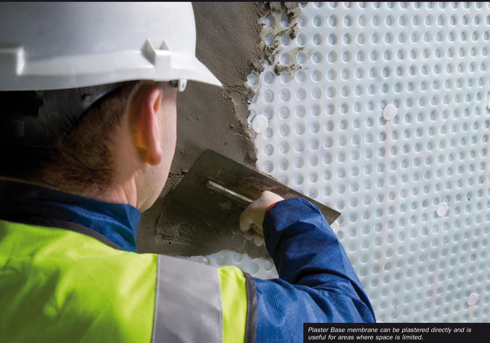
*Plaster Base membrane can be plastered directly and is useful for areas where space is limited.*
