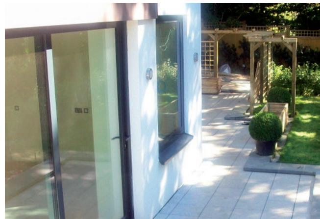
TT Vapour Membrane formed a waterproof layer below the terraces and landscaping
