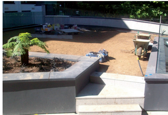
The residents' basement car park extends under soft and hard landscaping outside
